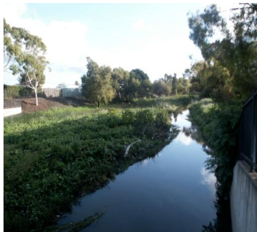
Wilmington Drain looking downstream from Lomita Boulevard
