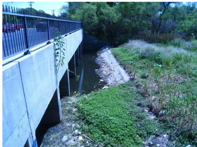
Figure C-6 Project 510 Outlet and Weir Downstream of PCH
